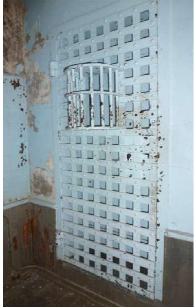
View of the entrance to the Sheriff's Office from inside the jail built in 1895. This doorway has two steel doors; the lattice iron door shown and a solid steel door immediately behind it. The "bird cage" like protrusion allowed the Sheriff to look into the jail proper without having to unlock the door itself. The cellblock, consisting of two four-bed cells, was designed by P.J. Pauly & Bro. of St. Louis, Missouri, which still builds jail cells and jail complexes today.
