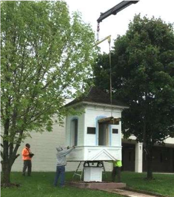
Durand Builders Service crew and crane lifting the bell tower from its concrete pad at the former Arkansas Elementary School.
